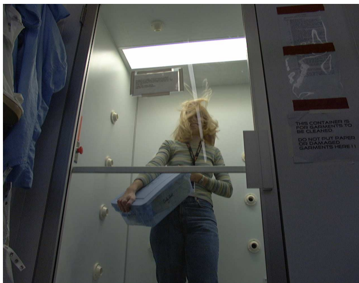
Figure A.1: When entering the cleanroom, an airshower greets you to blow off particles.
