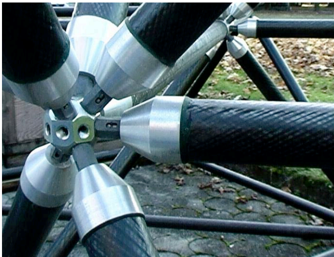
Mero Truss for MAGIC Primary Mirror
