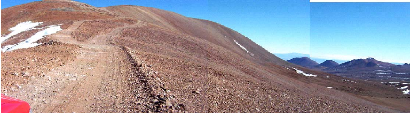
Figure10.2.3. Access Road to the Honar Ridge
